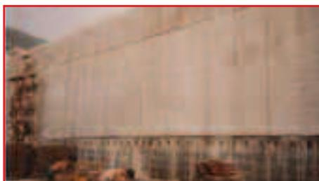
Early-age thermal cracking in a box section tunnel
