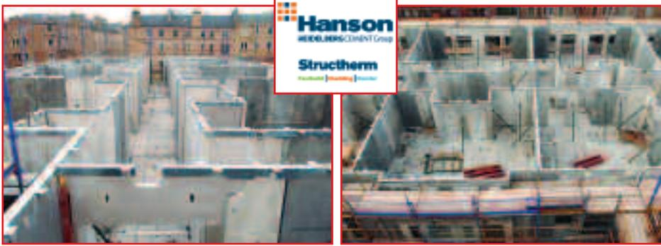
Use of Structherm's Fastbuild system on a confined inner city site
