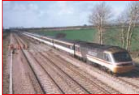
Poor compaction and steep slopes are characteristic of railway embankments
