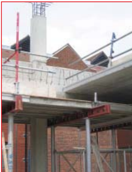
Hybrid concrete construction brings factory quality and efficiency improvements to site
