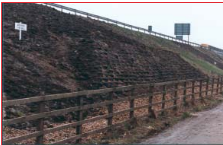
Tyre wall used to stabilise earthworks slope
