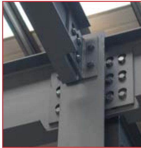
Quicon® Connection System being erected on a Dartford site.
