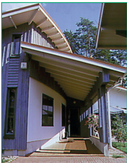
A house at Raisio, near Turku in Finland, constructed using straw-clay blocks, with lime render and timber cladding at first floor level. Architect: Teuvo Ranki. (Courtesy of Chris Morgan of Gaia Architects)
