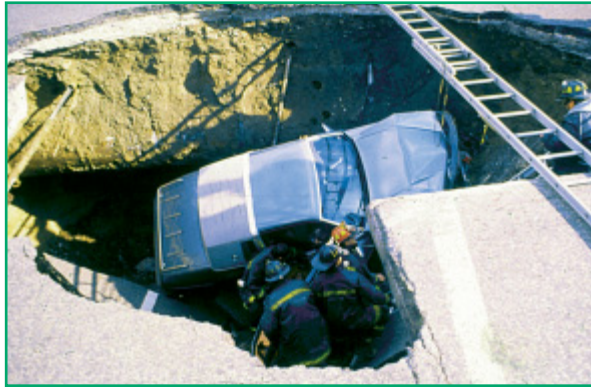
Neglected sewers can collapse with dramatic consequences. (Courtesy of Insituform Technologies®, Inc)
