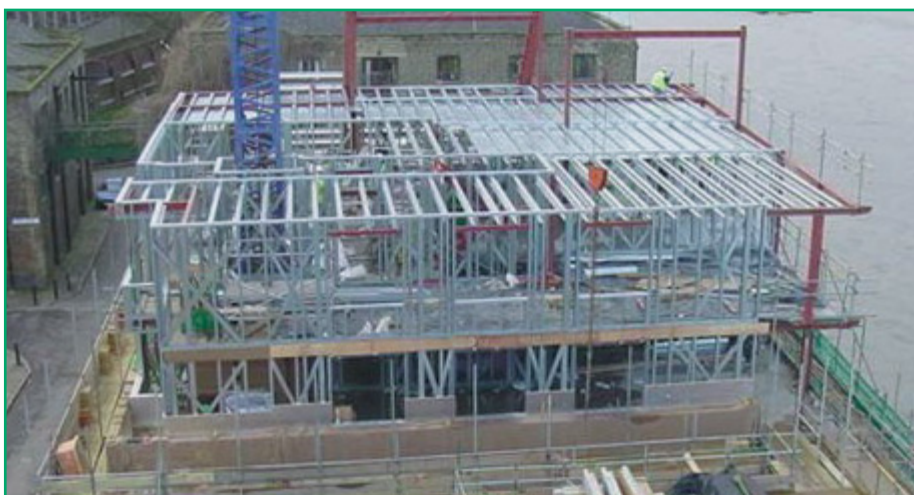
Light steel frame construction at Tunnel Wharf.
