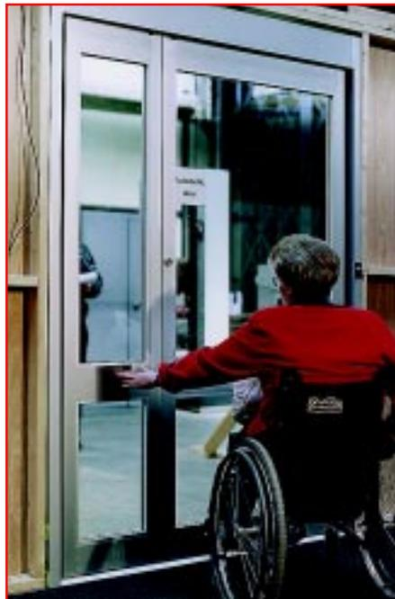
(Left) A metal and glass swing door used in laboratory tests: outward opening, with side panel, fully automated with electric lock, push plate internally and externally a coded key pad, closes automatically after a delay period, this was a commercial type door but could be used at the entrance to a communal block.
