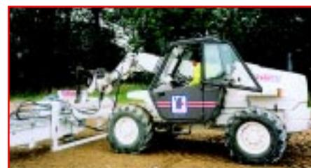
Equipment for inducing cracks in a cement-bound base.
